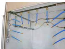
Multi-directional, non-metallic air and water lines.
